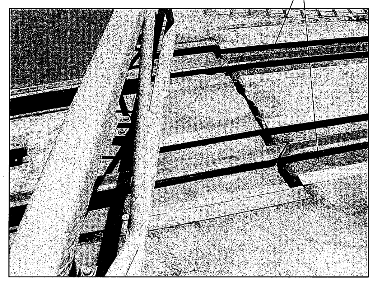
RSS RAIL BRIDGE BEARING AREA
